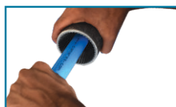
Step 3: Chamfering the Tubes
